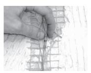
Step 3.13. Pull the heating wires together to overlap the heating elements of both leads. Lightly twist the elements together to better join them. Slide the solder tube over the twisted elements, centering the elements between the gray adhesive bands. If this is not done correctly, the elements may pull out and cause the splice to fail.
