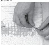
Step 4.3. Gently bend the cable at the score to break through the jacket all the way around the cable, then pull off
