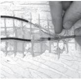
**Step 4.18.** At the other end of the jumper wires, slide a heating element solder tube over a heating wire or its jumper wire, whichever is easier for you to position the tube out of the way and allow for easy access to the ends of the wires. REPEAT Steps 4.14 through 4.17 to complete the heating element jumper wire connections.
