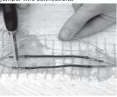
**Step 4.19.** If necessary, cut the ground jumper wire shorter so that it overlaps the ends of the ground wires by about 1/2" to 3/4".
