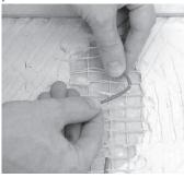
**Step 3.3.** Gently bend the cable at the score to break through the jacket all the way around the cable, then pull off the slug
