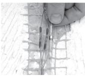
Step 3.16. Slide a ground solder tube onto the longer ground wire. Overlap the ground wires and twist them to help hold them together. Slide the ground solder tube over the twisted ground connection centering the connection under the ring of solder.
