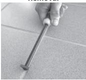
Step 2.1. If not done so already, carefully remove the tile/stone/marble floor covering over the damaged cable area. Removal of the grout around the affected tile(s) must be done with a blunt instrument such as a hand-held grout-removal tool. DO NOT USE A KNIFE! Gently break out the tile with a small hammer, removing the fragments as the tile is broken up.
