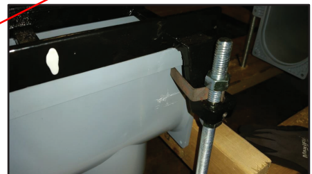
The Clip on 6" DI Frame Engages The Channel Against The Side Underneath The Lip
