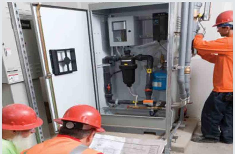
control station, the treatment station, and the pressure booster pack all in one; the skid containing the Rainset™ also includes monitoring, pumping, and cleaning controls. The NACO Border Patrol expects to collect nearly half a million gallons of rainwater each year which it will use for flushing toilets and irrigating outdoor plants.
