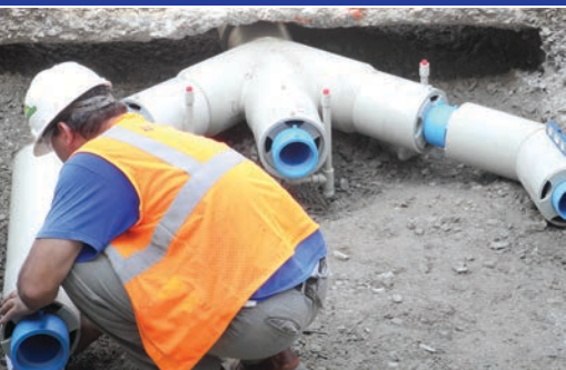
Double-containment piping systems
