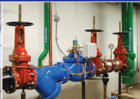
Flood protection shutdown valves
