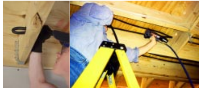
Onix is easy to work with in Staple-up jobs because of its flexibility. It's great for retrofitting, too.
