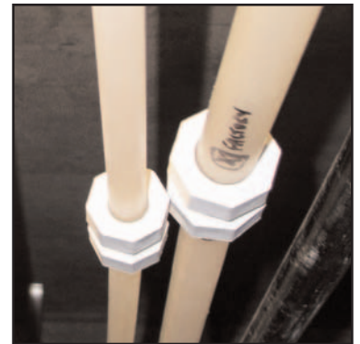
Fig. 4. Pipe installed crooked and improperly supported.
