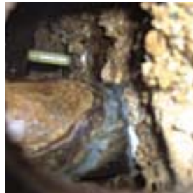
Large deposits of hard scale constrict water flow of this hotel plumbing system.
