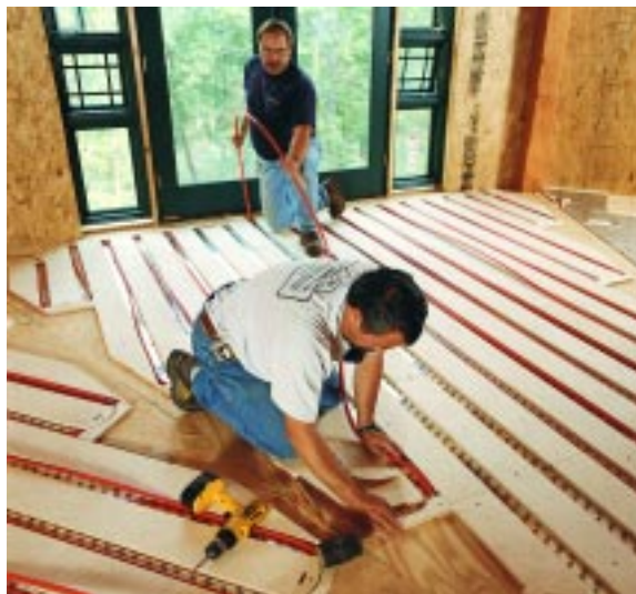
RadiantPEX in a residential SubRay™-heated floor.
