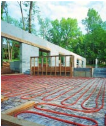
RadiantPEX in a residential slab heating system.
