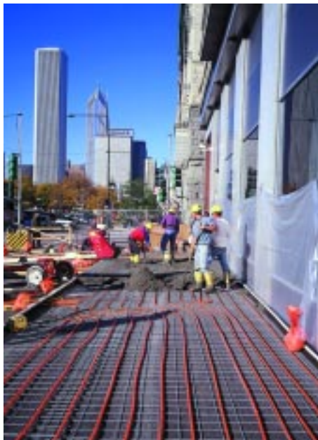
RadiantPEX in a commercial snowmelting system.
