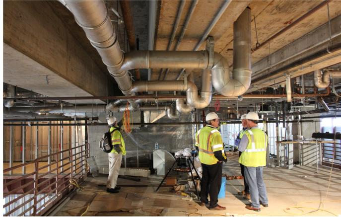
*“The project turned to stainless steel because of its light weight, corrosion resistance, tolerance to high temperatures and ready availability.”*
