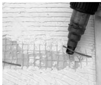
Step 4.4. Use the heat gun (set to HI temperature, about 1000°F) and move the gun back and forth under the jacket slug for about 3 to 4 seconds until it starts to loosen and slightly shrinks at the ends.
