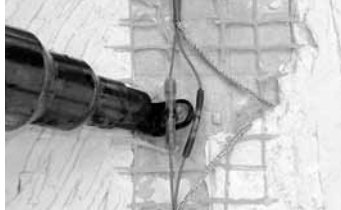
Step 3.15. REPEAT Steps 3.12 through 3.14 for the other heating wire.
