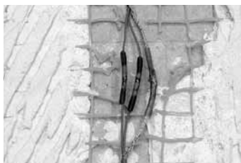
Step 3.18. The connection should now be complete and ready to test. Go to Step 5.1 under "Testing the Repair."
