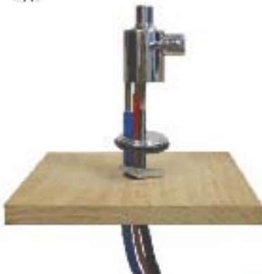
Feed attached tubing and toggle bolt through counter top.
