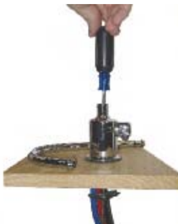
Set toggle bolt with Phillips head screwdriver from above the counter top.
