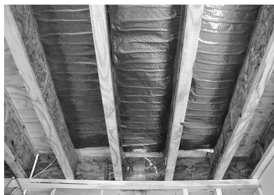
Watts Radiant UnderFloor - multiple joist bays
