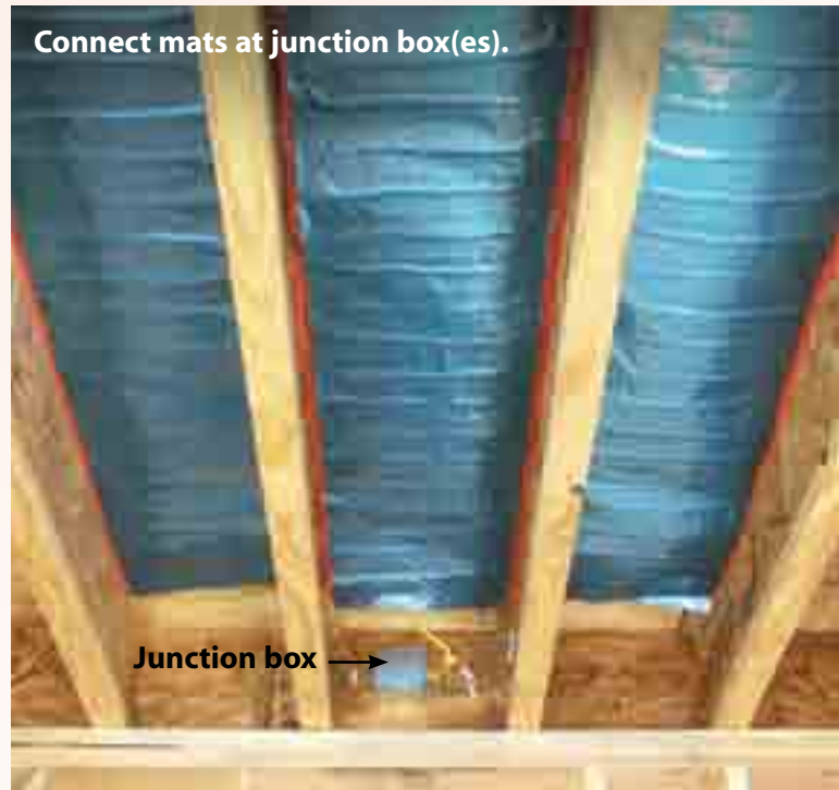
Install insulation.
