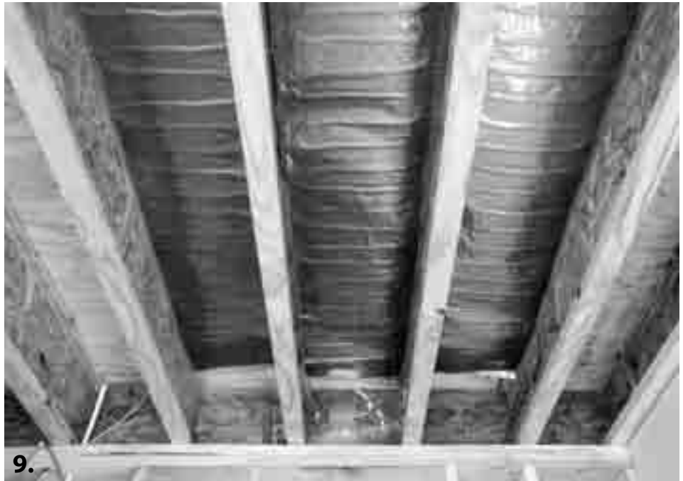
6. At the other end of the mat, place a nail into the joist at 2" below the sub-floor. Hang the fiber mesh of the mat onto the nail. This will make it much easier to staple the rest of the mat.
