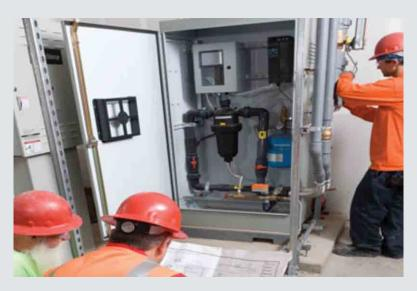
control station, the treatment station, and the pressure booster pack all in one; the skid containing the Rainset<sup>™</sup> also includes monitoring, pumping, and cleaning controls. The NACO Border Patrol expects to collect nearly half a million gallons of rainwater each year which it will use for flushing toilets and irrigating outdoor plants.
